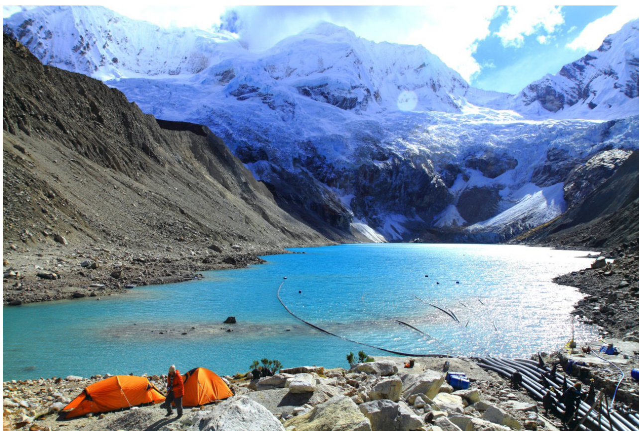
Figure 5. Palcaraju Glacier and Lake Palcacocha in 2013, with siphons removing water to reduce the possibility of a GLOF. Photo: Paribesch Pradhan, from the Glacier Photograph Collection, National Snow and Ice Data Center, Boulder, Colorado, USA.
